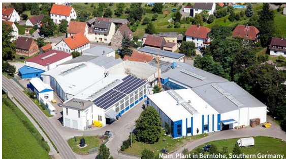
Main Plant in Bernlohe, Southern Germany
